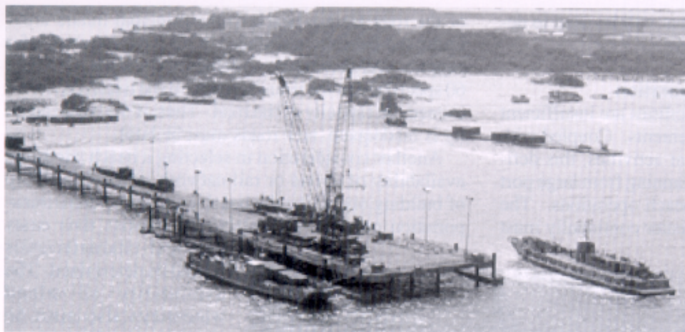
□ A crane lifts equipment from a vessel positioned alongside an elevated causeway system.
